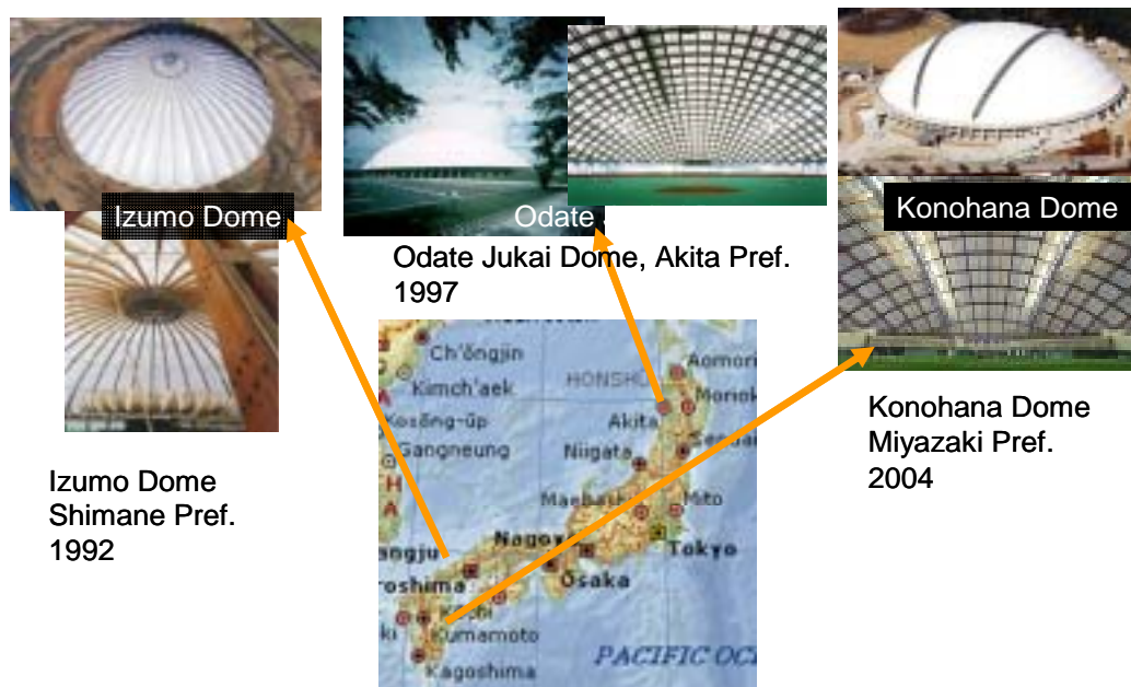
Figure 3 Large Scale Wooden Frame Domes in Japan ( Photos are provided by the City Hall of Izumo City Takenaka Corporation/ Miyazaki Wood Techno Co.,Ltd.)
